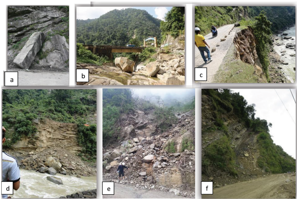
Fig. 5. Rock slope failure problem (a, b), Block failure type (c, d), Slope scar collapse and Debris flow (e & f).
